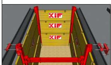
23. Installation of a upper water by means of a beam girder with a large cross-section.
