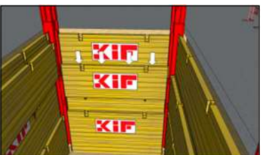
17. Then, Top panels are then snapped onto the base panels at the bottom of the excavation (in the inner rail)..
