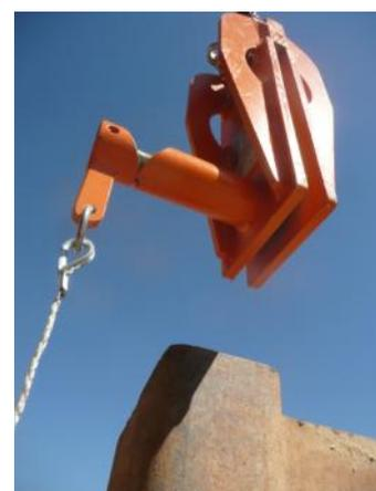
The clamp releases the sheet pile.
