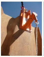
The clamp releases the sheet pile.
