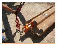
The sheet pile fixed, secure handling can be done.
